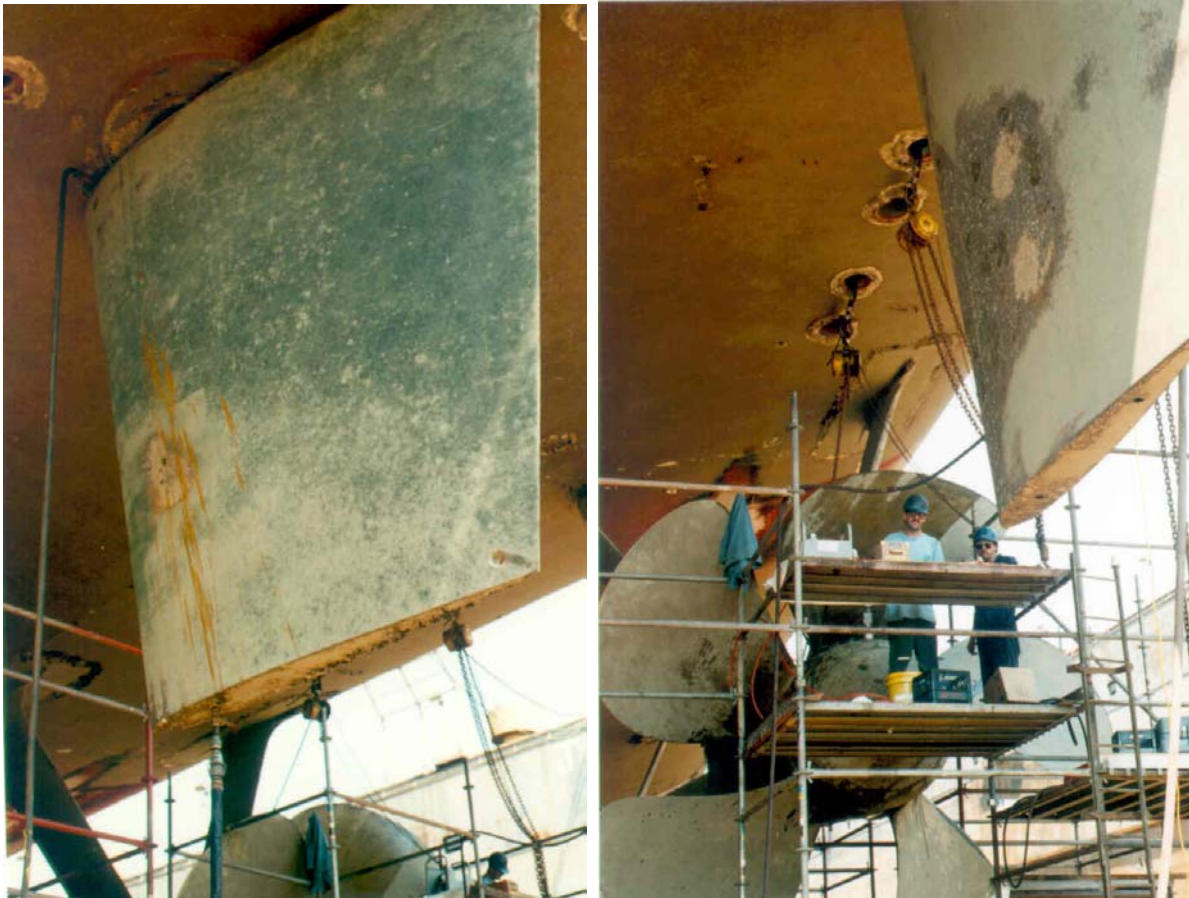
Photographs of rudder cavitation damage.
