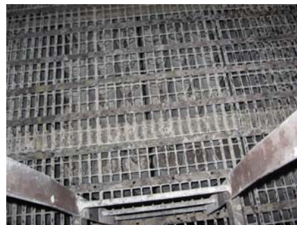
Top of the Compartment Bags are suspended from springs attached to the grate.
