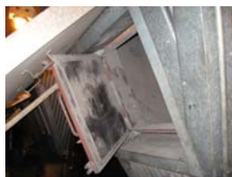
Front of Hopper Door is open in preparation for the annual inspection
