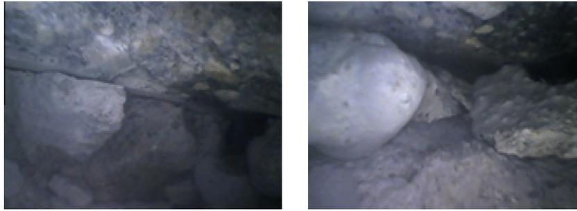
Fig. 5. Sample photos of borescoping showing the void positions within the concrete blocks.
