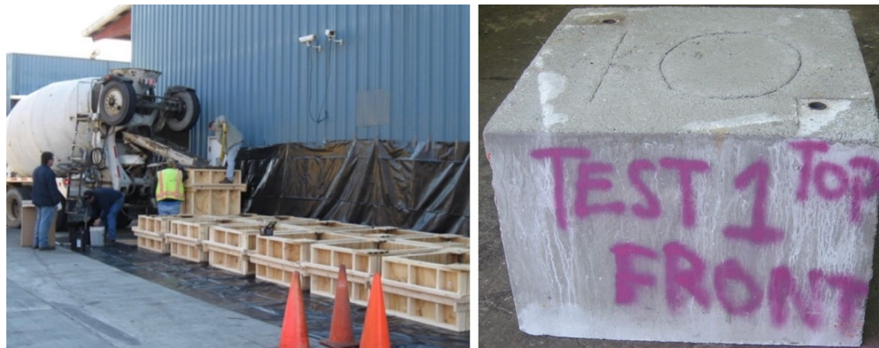
Fig. 4 Pictures of pouring concrete blocks and cured testing samples
