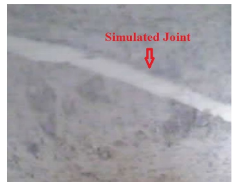
c A simulated joint in borescoping
