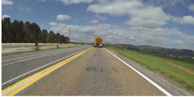
Figure 5.6. Lane lines being painted at the Larson Transportation Institute test track
